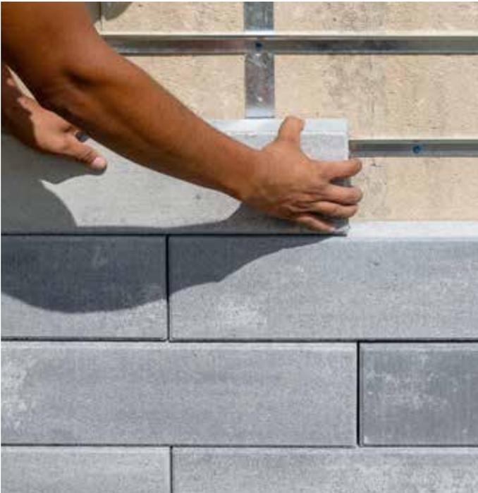
The U-Cara Wall Mount System allows you to put the finishing touches on your project by cladding existing structures like unsightly exposed foundation areas or concrete steps with U-Cara fascia panels.
